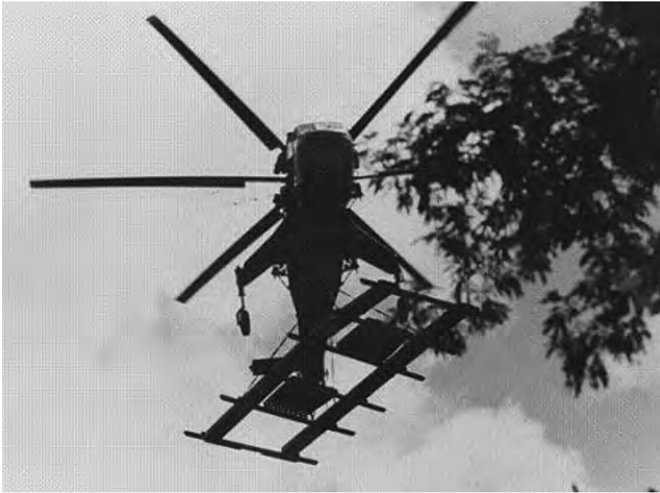
A CH-54 Flying Crane transports fixed-span bridging during the Cambodian incursion.
